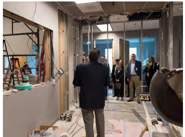
2016: Brian inspects the progress on his state-of-the-art podcast studio.
